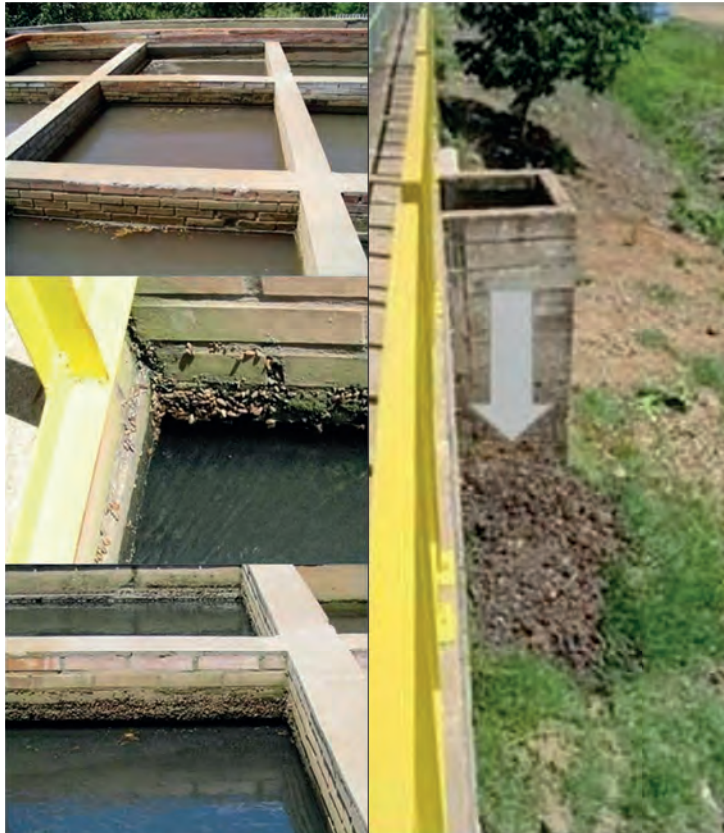
Figure 16. Corsan station, in Rio Grande do Sul, showing the colonization of tanks by the golden mussel and the residue removed. Photo: MCD Mansur.
