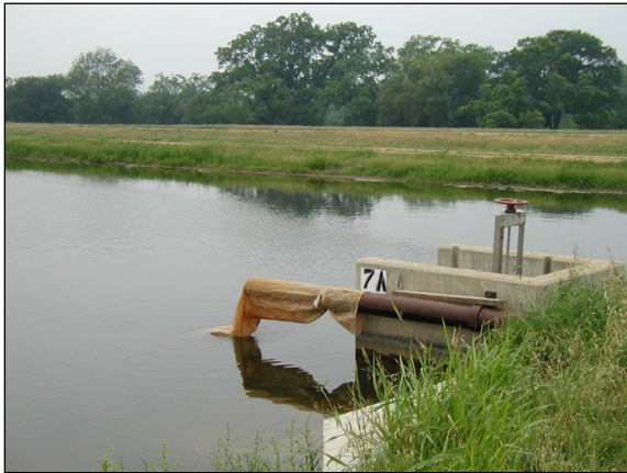
Filtering “sock” on pond water supply line. Photo Credit: Bob Pitman & Robert Lindsey, USFWS
