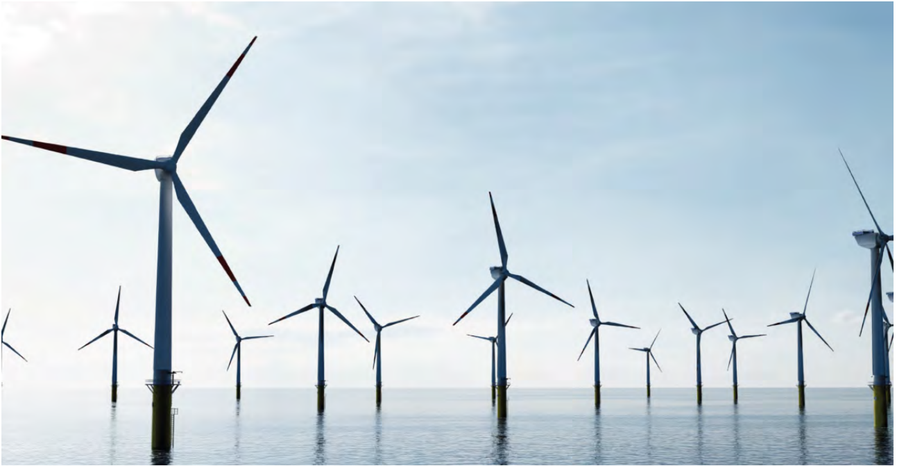
Figure 4.30 Fixed offshore wind farm Image.. Source: Hywind Scotland.
