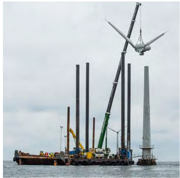
Figure 4.37 Vindeby (Denmark) decommissioning in 2016. Source: Orsted.
