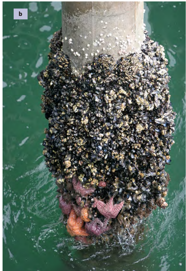
Figure 2.4 a) A concrete marine structure with severe biofouling. Source: Vorathep Muthuwan /Shutterstock.com; b) Mussels on a pier pillar. Source: Mikeledray/Shutterstock.com
