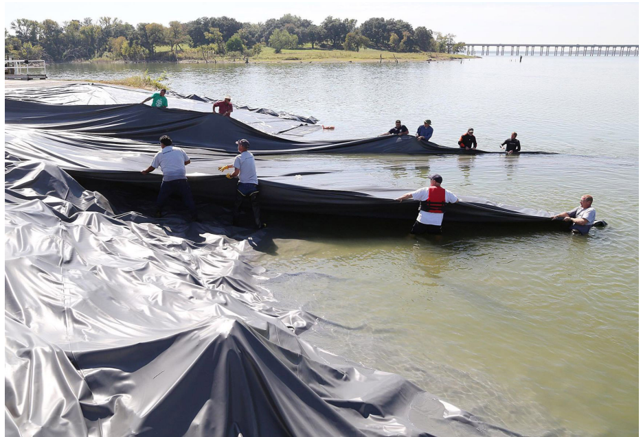
Figure 1. Placement of PVC sheet benthic barrier for zebra mussel eradication efforts. Photograph by Texas Parks and Wildlife Department.
