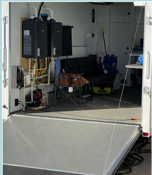
Figure 2. Mobile inspection station with a built in on-demand decontamination unit at Loma, Colorado Port of Entry. Top: Inspection trailer. Above: On-demand hot water unit mounted inside inspection trailer.
